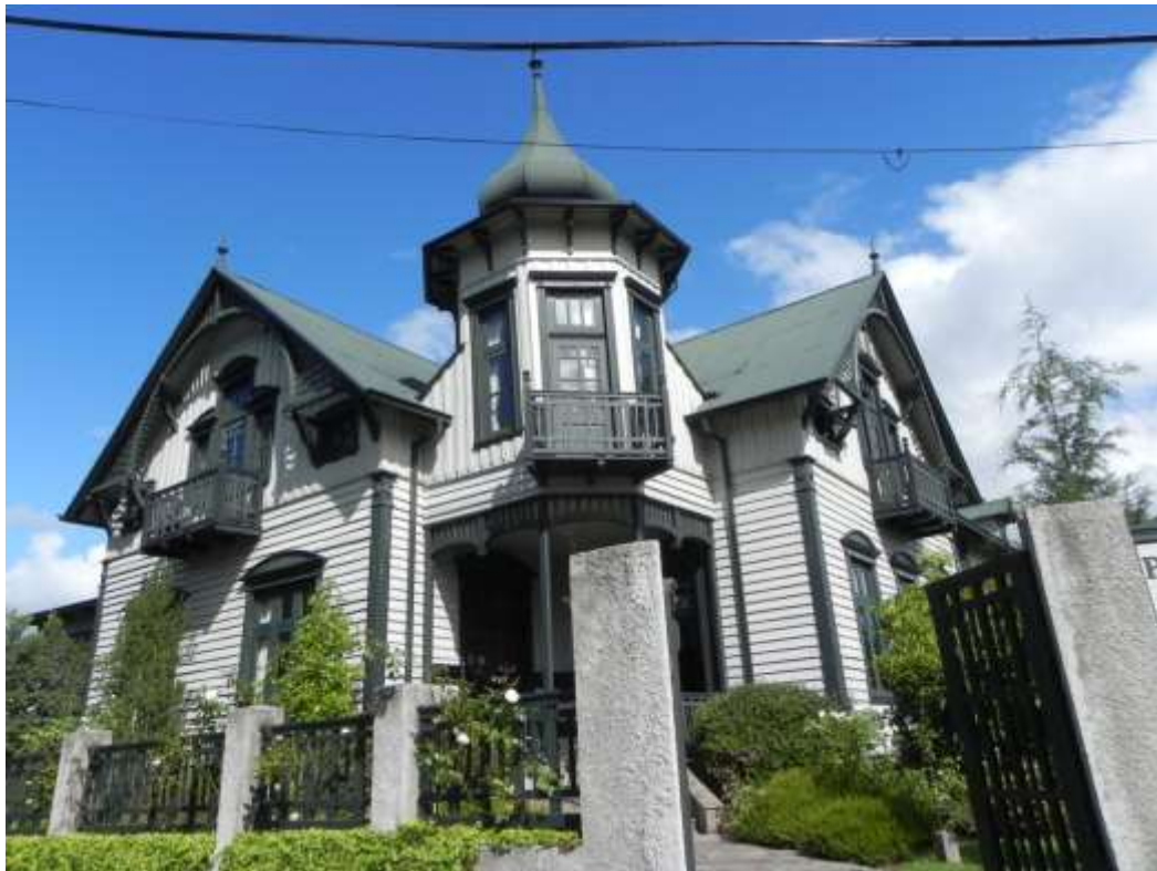
Casa Kuschel in Puerto Varas
